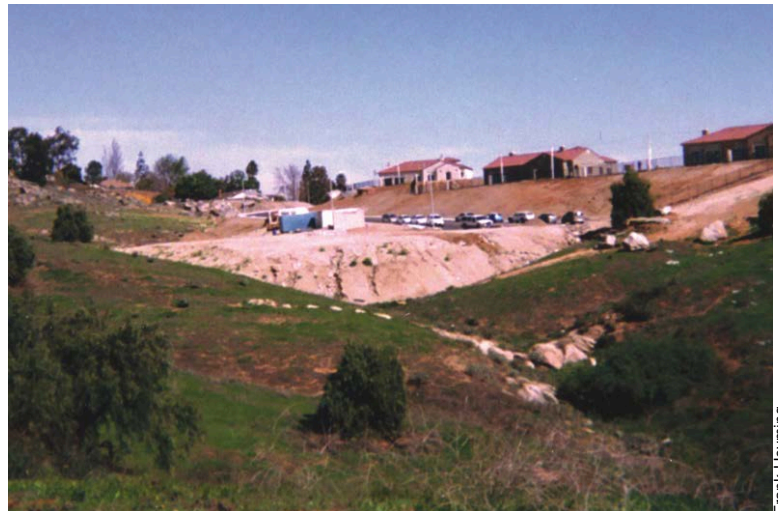
A house pad fills an important tributary to a waterway.
